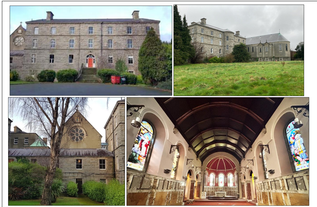
Figure 5.2: Images of Tabor House (Top) and the Chapel (Bottom) to be reused within the development
