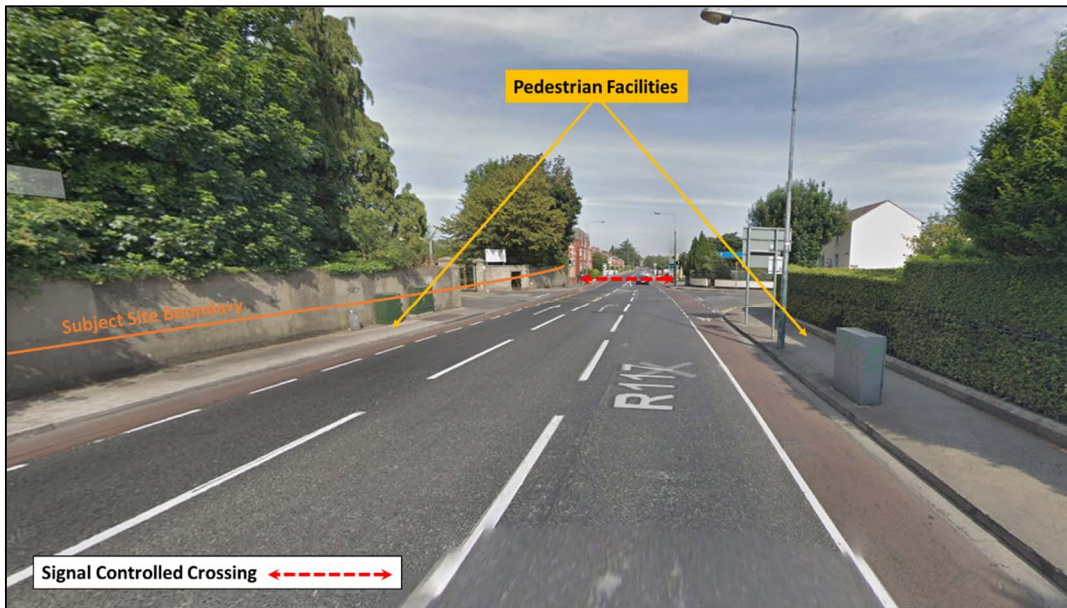
Figure 2-6: Existing Pedestrian Facilities along Sandford Road
