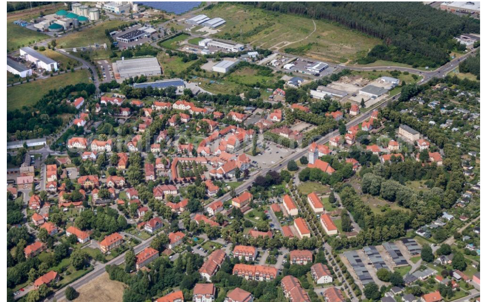
Example of residential development in parkland - Marga in Senftenberg Brieske Garden City, Brandenburg
