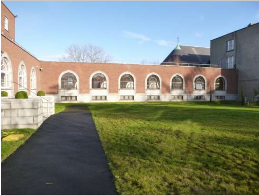
CENTRAL SECTION OF SOUTHERN BOUNDARY – LOOKING NORTH
