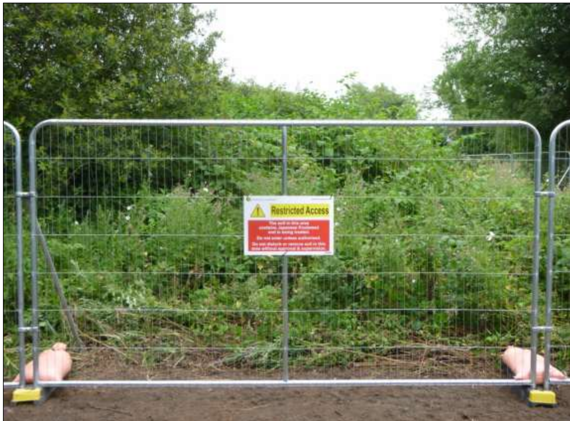
SAMPLE FENCING 2 – HEAVY DUTY HERAS FENCING
