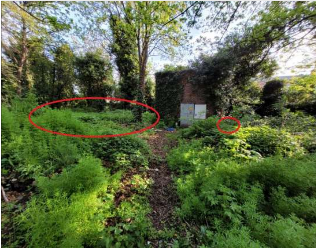
LOCATION OF STANDS IN RELATION TO THE E.S.B. SUB-STATION
