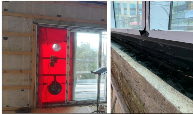
Figure 3: Air Tightness Testing Examples
