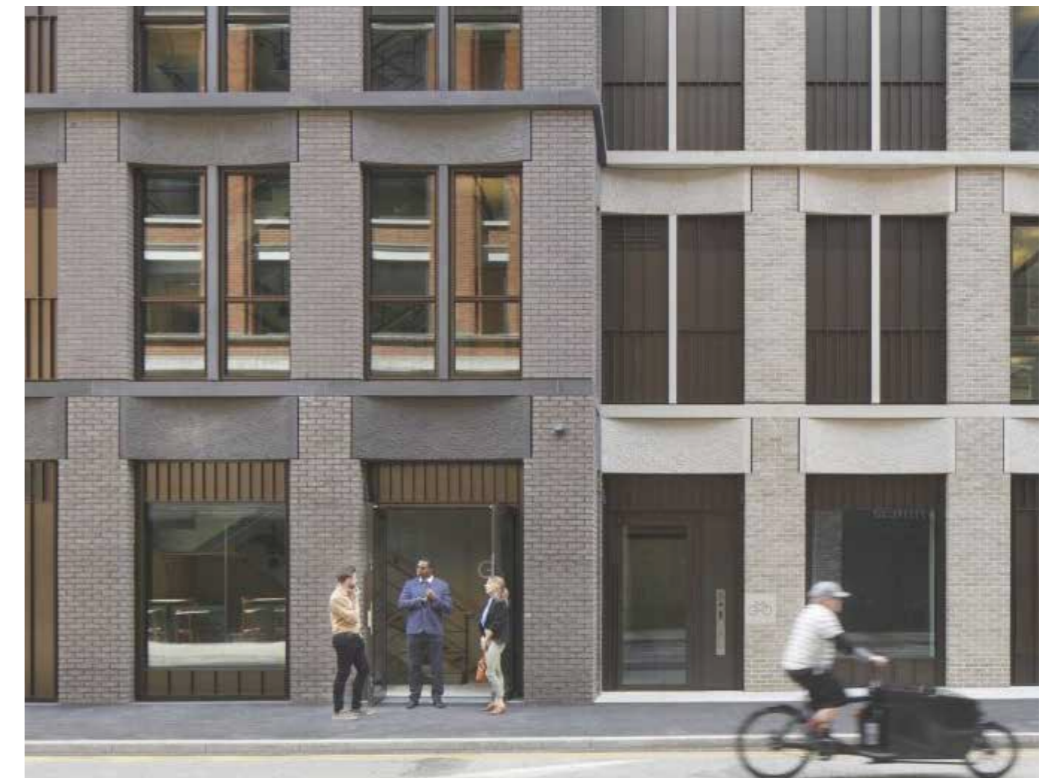
Main: North East corner of Block C facade Above: Brick facade with pre-cast concrete horizontal band & window sill - Morris & Co Architects
