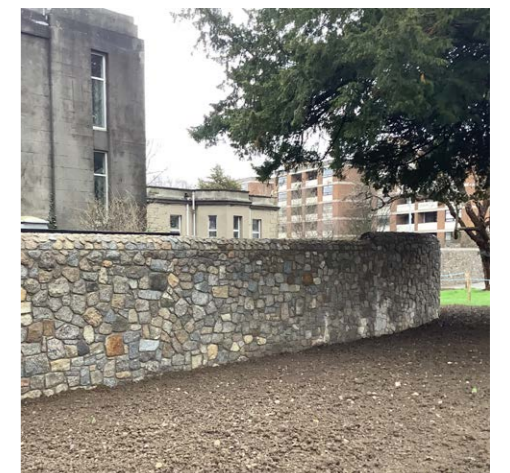
Perimeter Stone Wall to South
