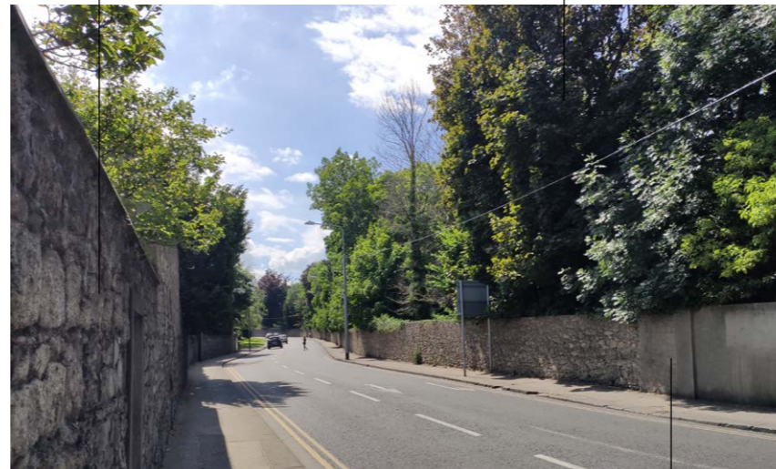
2 View looking South along Milltown Road
