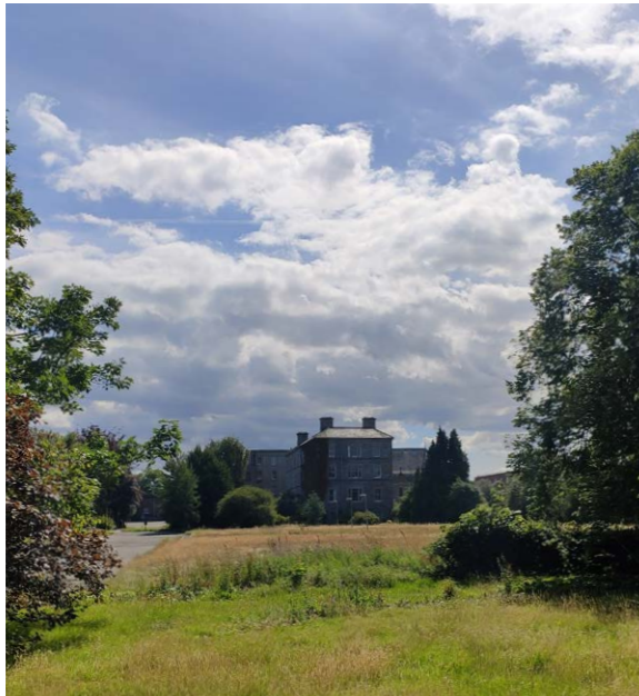
3 View South of Tabor House from Entrance
