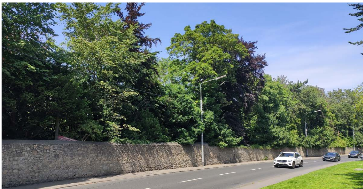
4 Tree Belt + Perimeter Stone Wall from Milltown Road
