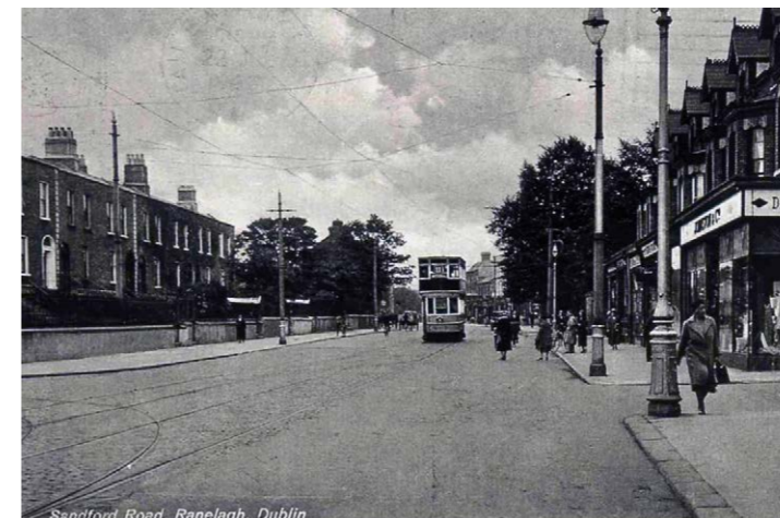
③ Junction at Chelmsford Road
