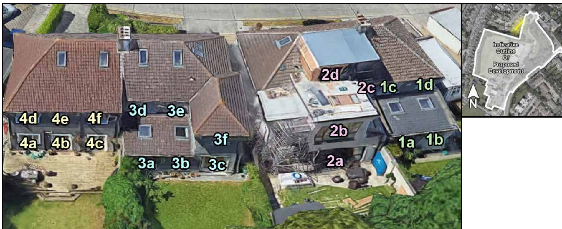
Fig. 3.2: Highlighted areas indicate the position of assessed windows (L), Aerial view of assessed location (R)
