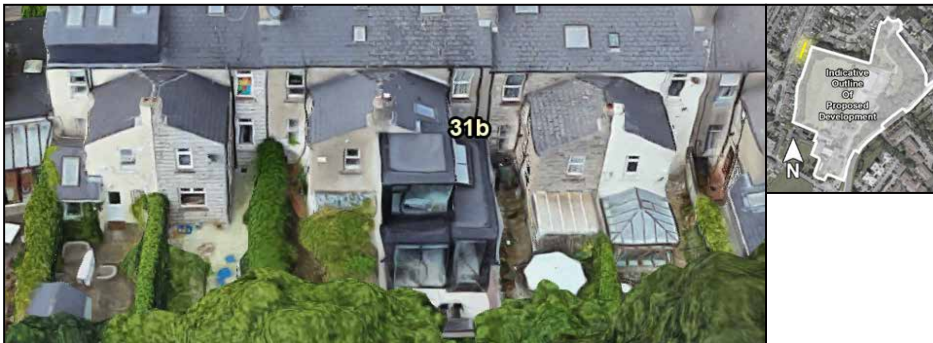
Fig. 3.7: Highlighted areas indicate the position of assessed windows (L), Aerial view of assessed location (R)
