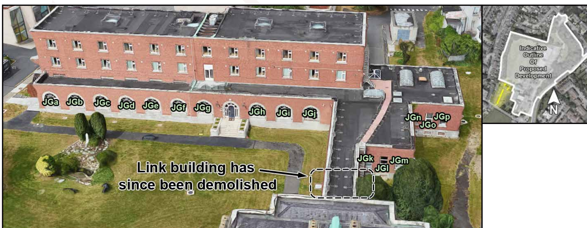
Fig. 3.3: Highlighted areas indicate the position of assessed windows (L), Aerial view of assessed location (R)
