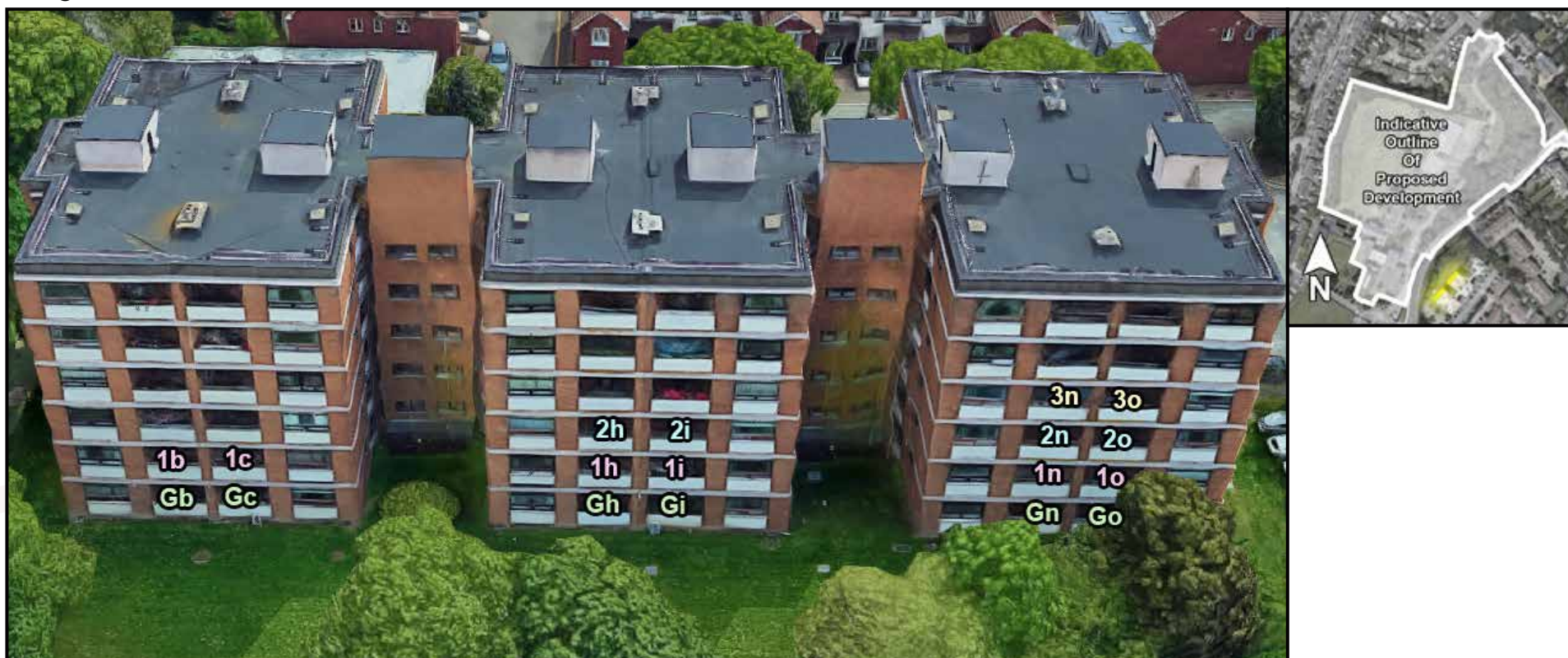
Fig. 3.1: Highlighted areas indicate the position of windows that are impacted as a result of existing balconies (L), Aerial view of assessed location (R)
