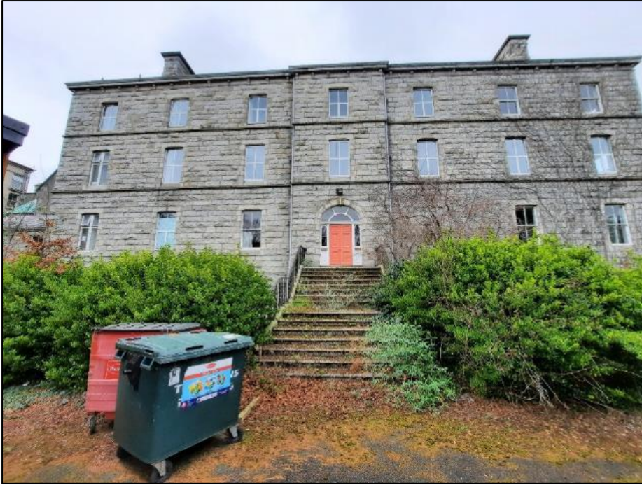
Figure 8.30: Tabor House (Source: DNV).
