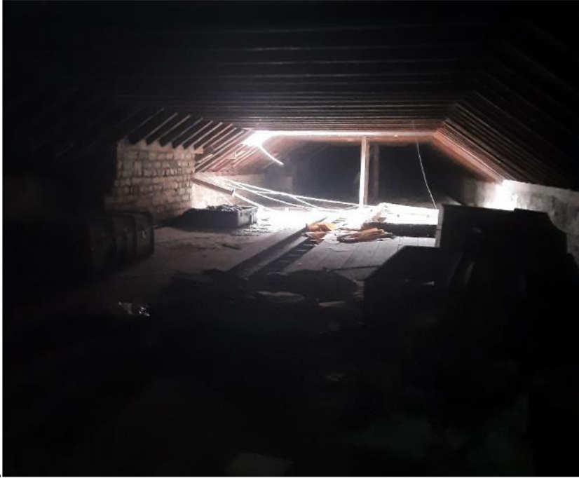
Figure 8.32: Image of the attic of Tabor House with light-spill from skylight evident (Source: DNV).
