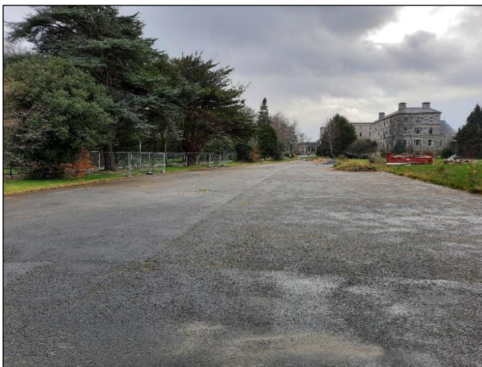
Figure 8.14: Buildings and artificial surfaces (BL3) viewed from the north (Source: DNV).
