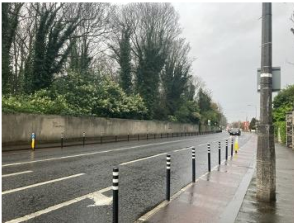
Plate 7.3.33: Section of boundary wall at junction of Milltown and Sandford Roads, due northwest which was replaced with blockwork in past realignment of the junction
