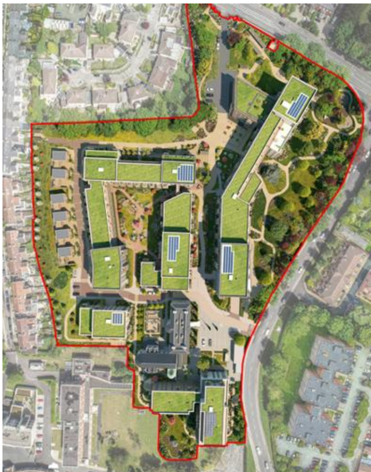
Figure 7.1.3: Aerial view of development site as proposed (Source: OMP Design Statement)
