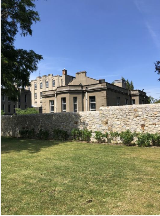
Plate 7.3.34: Contained boundary, enclosing extant building range
