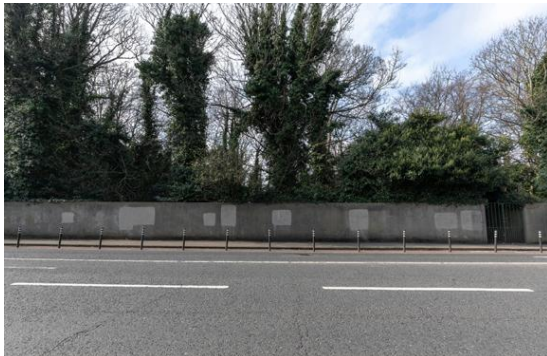
Figure 7.5.16: Viewpoint V3- existing Replacement section of boundary wall along Milltown Road
