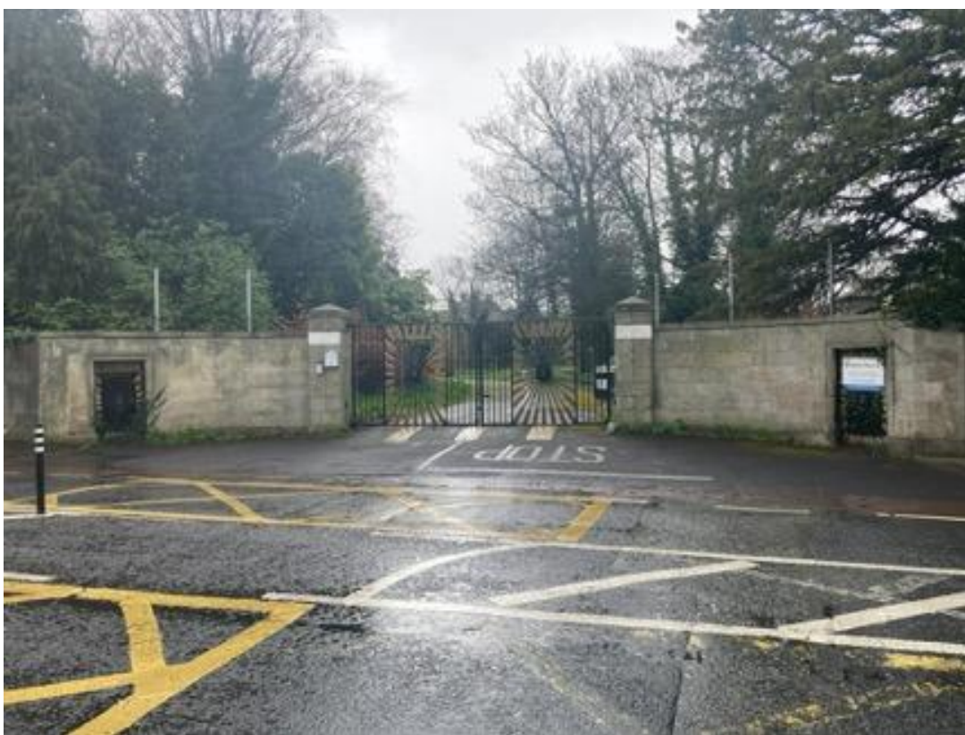
Plate 7.3.29: Gated entrance on Sandford Road
