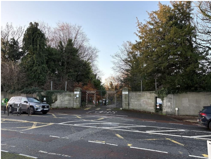
Plate 7.3.3: Sandford Road entrance to the development site
