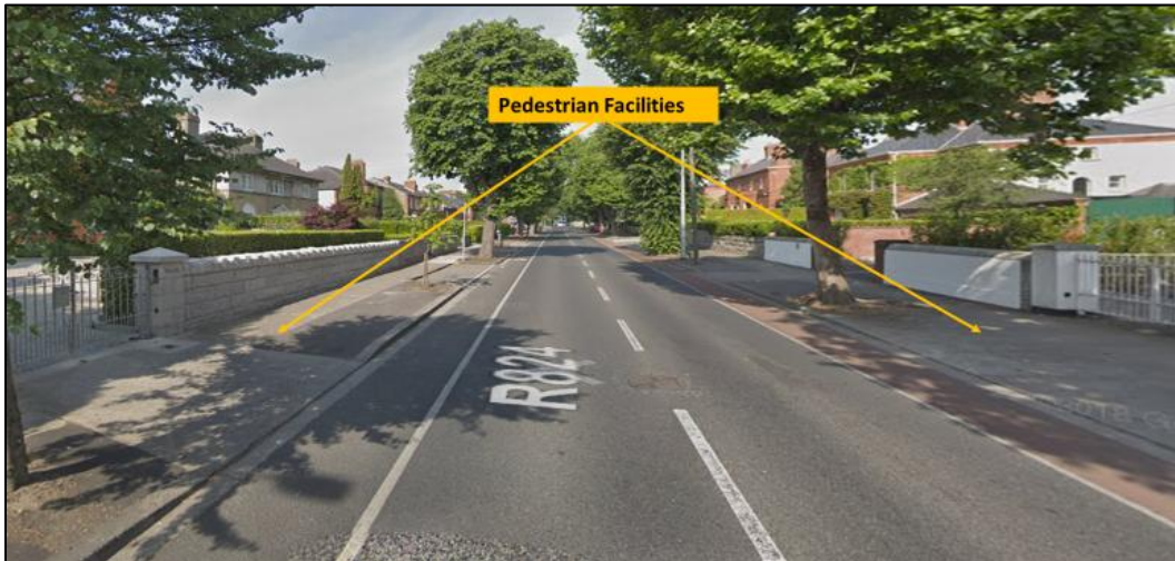
Figure 15.7: Existing Pedestrian Facilities along R824 Eglinton Road
