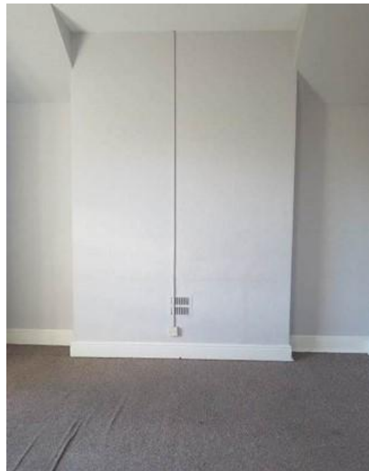
Plate 261: Example of removed chimney piece to typical bedroom.
