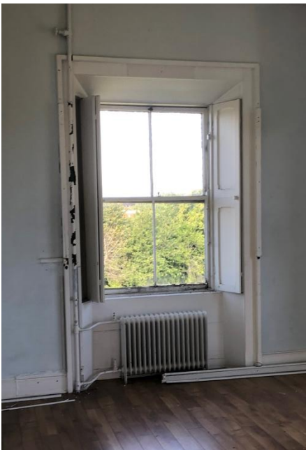
Plate 260: Detail of tripartite sash window.
