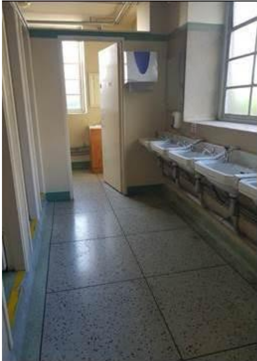
Plate 343: Toilets within the same area
