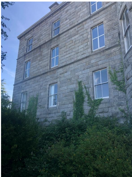
Plate 29: North east gable elevation of Tabor House
