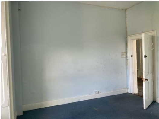
Plate 268: Typical upper floor accommodation. Original four paneled door and architrave.
