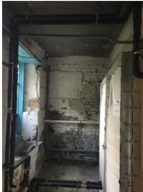
Plate 98: View east in same room
