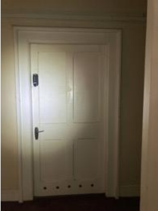
Plate 306: Typical panelled door and architrave at basement level.
