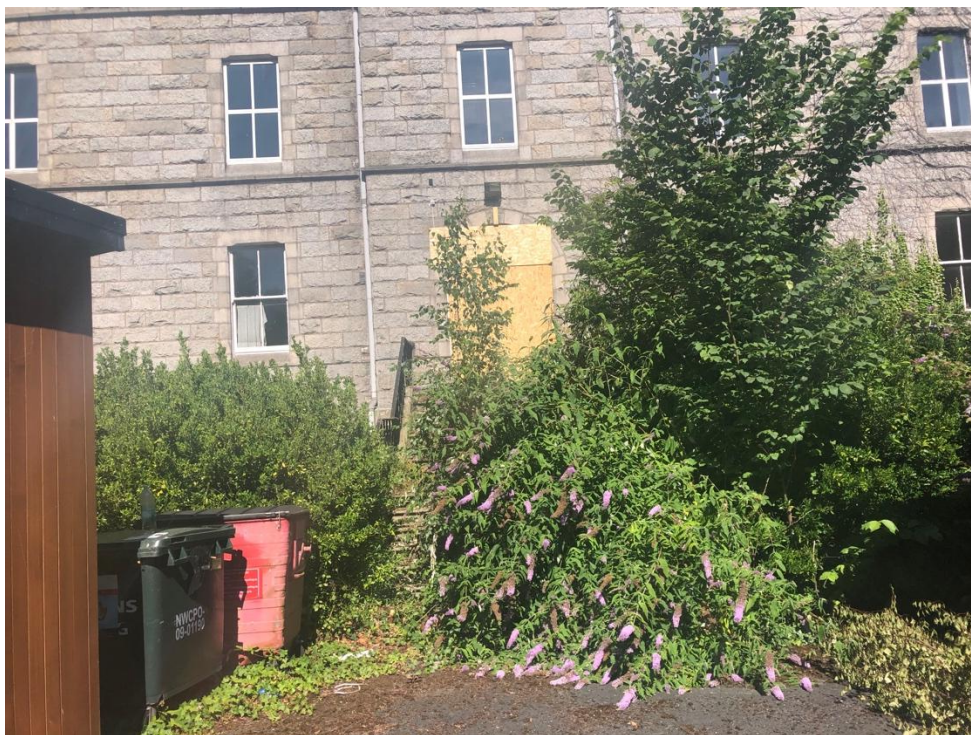
Plate 23: Original panelled front door with fanlight and granite steps to Tabor House
