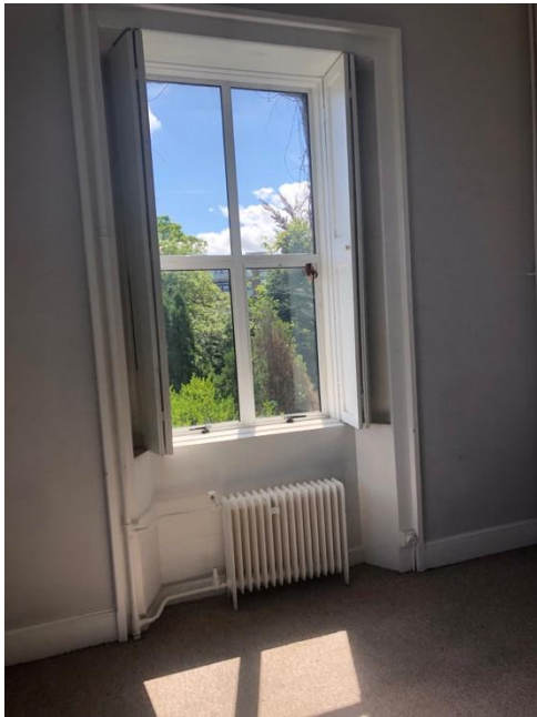
Plate 246: Dormitory facing south east, original window-box with contemporary uPVC window.
