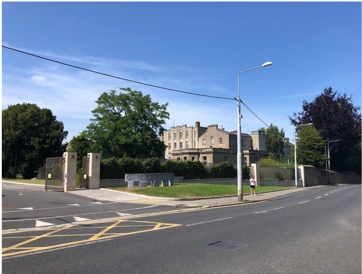
Plate 55: East elevation of the Archive (built 1938) in background (with south side of Finlay wing in view)
