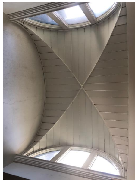
Plate 321: Clerestory light above boarded groin vault
