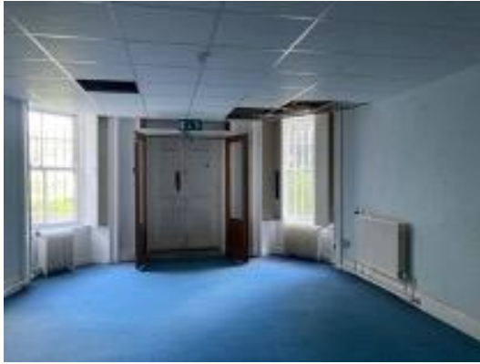
Plate 234: Lower ground floor entry to rear (north) elevation within rounded bay. Later suspended ceiling.
