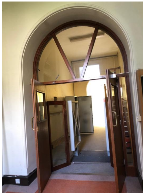
Plate 156: Round headed opening to lobby affording access to former domestic Chapel.
