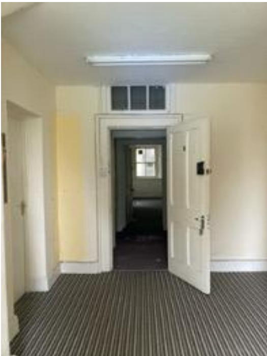
Plate 308: Panelled door with transom light over.
