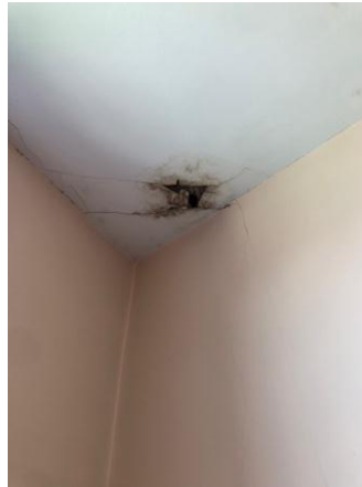
Plate 161: A typical dormitory. Exposed services.
