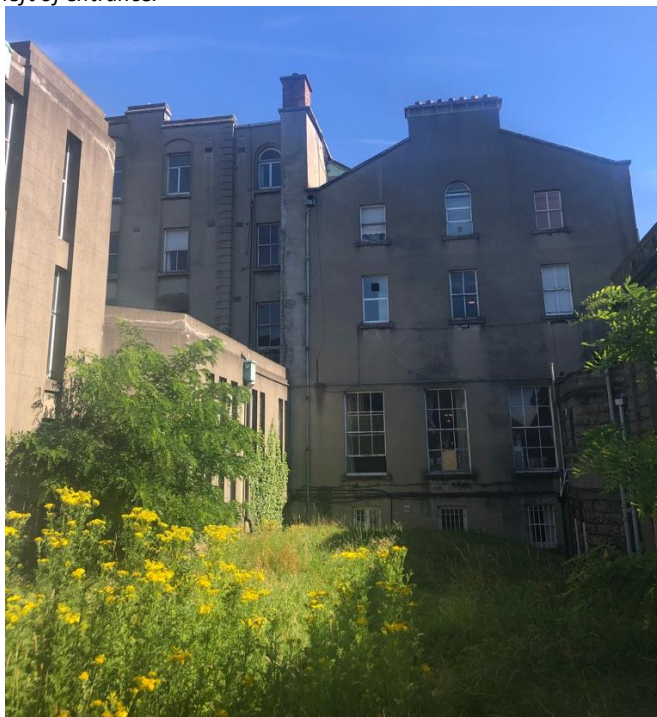
Plate 10: View on south-west elevation of MPH, positioned between the Archive (left) and the Finlay wing (right).
