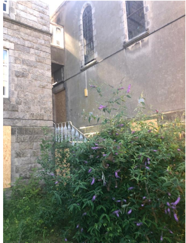
Plate 32: Cast iron balustrade on stairs to 1st floor
