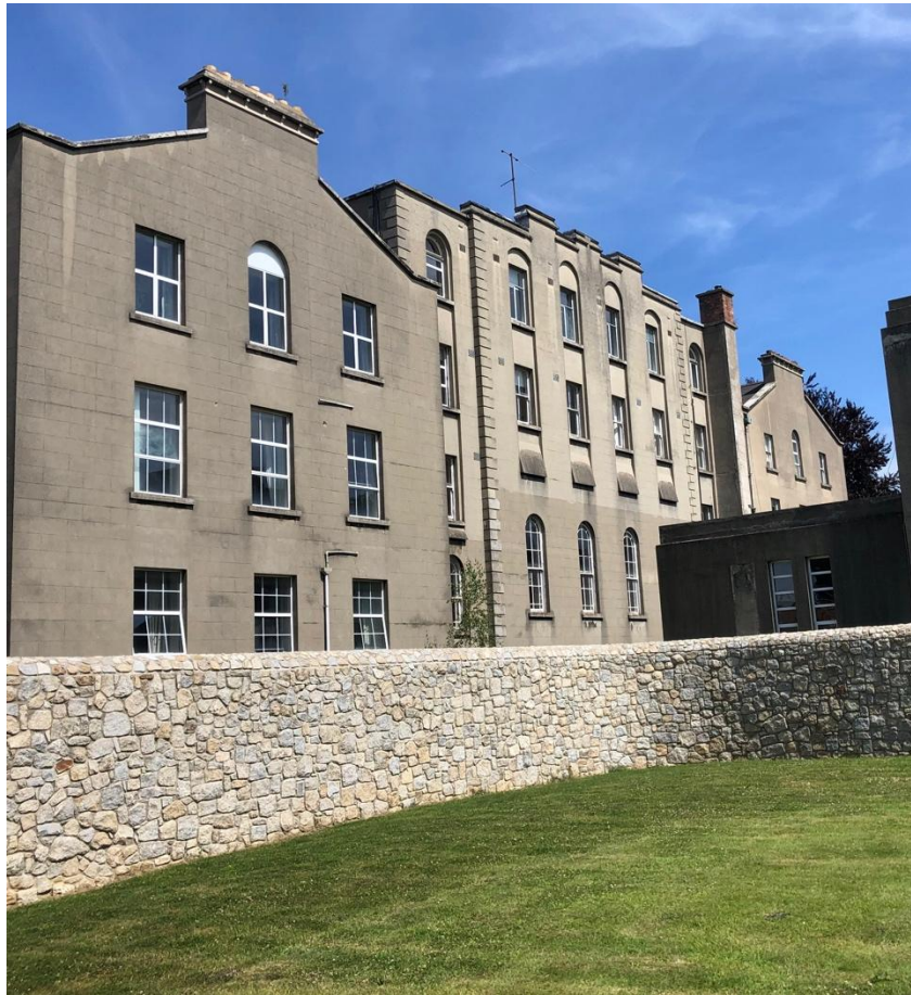
Plate 20: South-west elevation of the rear extension to MPH, with projecting gable to match that on eastern end, and new boundary wall in foreground
