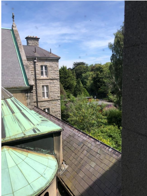
Plate 44: Copper Roof of sacristy, building D2
