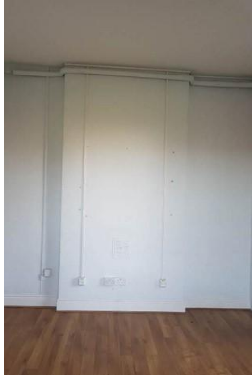
Plate 215: Chimneypiece removed. Contemporary services surface mounted throughout.
