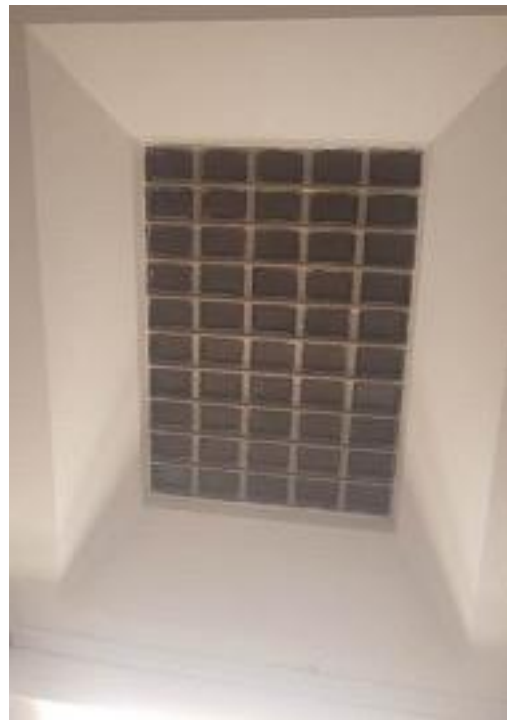
Plate 181: Example of cast iron rooflight at 2 nd floor level
