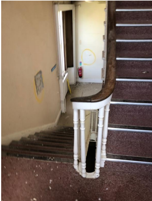
Plate 184: Painted stair to rear of block
