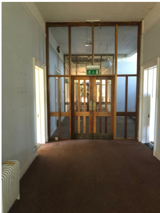
Plate 204: Cross-corridor fire screens, original molded architraves to paneled doors either side of corridor.
