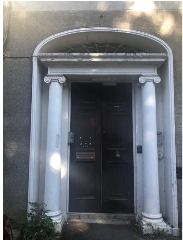
Plate 2: Main entrance to Milltown Park House with original ionic columns and cobweb fanlight over
