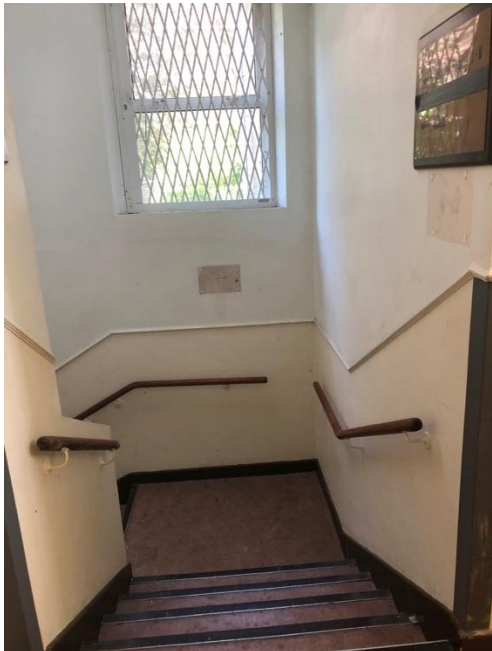
Plate 315: Contemporary stairs to basement
