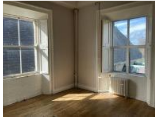
Plate 275: Original window joinery, with contemporary uPVC window frame in north elevation.
