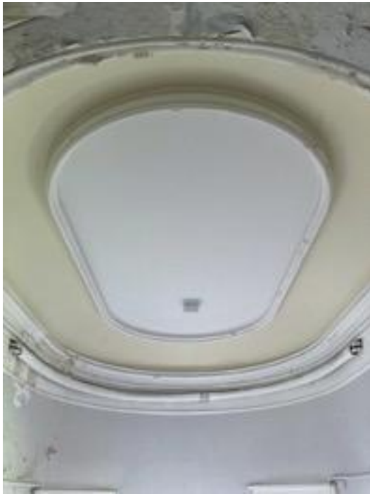
Plate 191: Coffered ceiling and moulded cornice within main stairwell.
