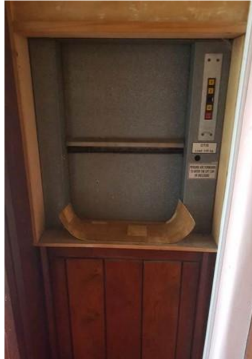
Plate 227: Dumb waiter from kitchen to dining area
