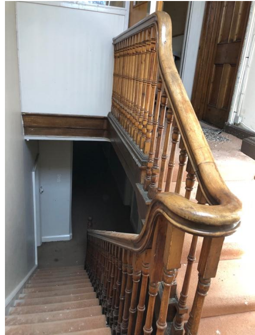
Plate 171: Detail of stair, hardwood handrail with swan-neck detail at landing.
