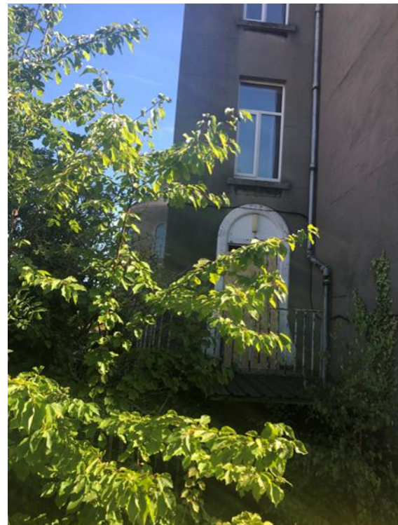
Plate 17: Panelled door to rear entrance of rear extension, late 19 th century
