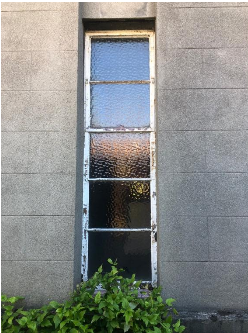
Plate 369: Early 20 th century steel windows with casement openings.
