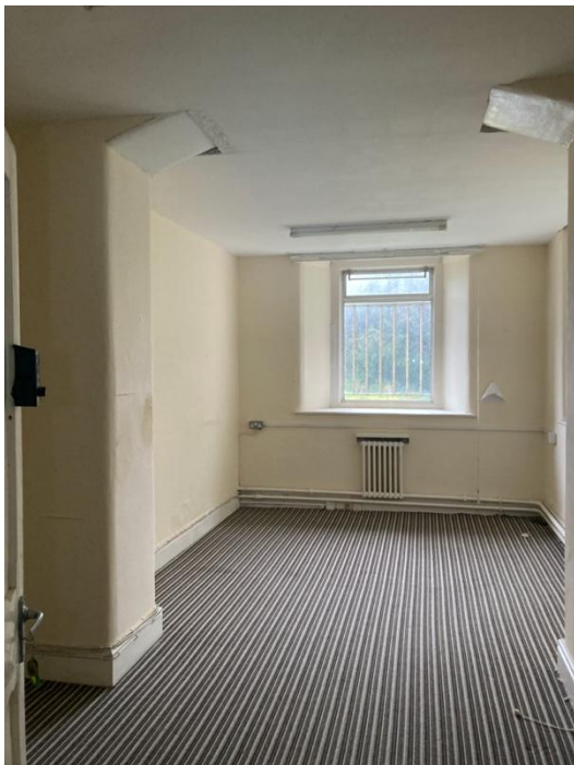
Plate 300: Lowered ceiling. Arched openings supporting columns in Chapel above. Contemporary windows. No decorative plasterwork.
