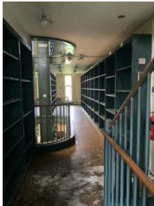
Plate 362: View towards central atrium
