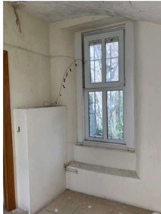
Plate 231: Contemporary uPVC window on lower ground floor. Beneath main entrance.
