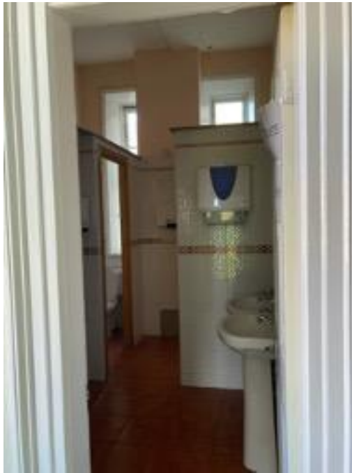
Plate 140: Toilet block within 1 st floor level
