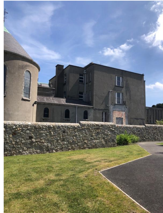
Plate 39: Rear of linking building with boundary of neighbouring property.
