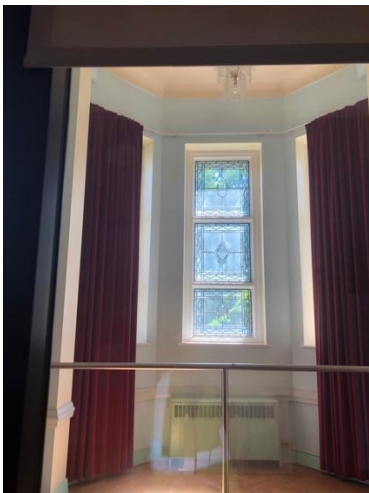
Plate 335: Chamfered bay window with leaded windows.
