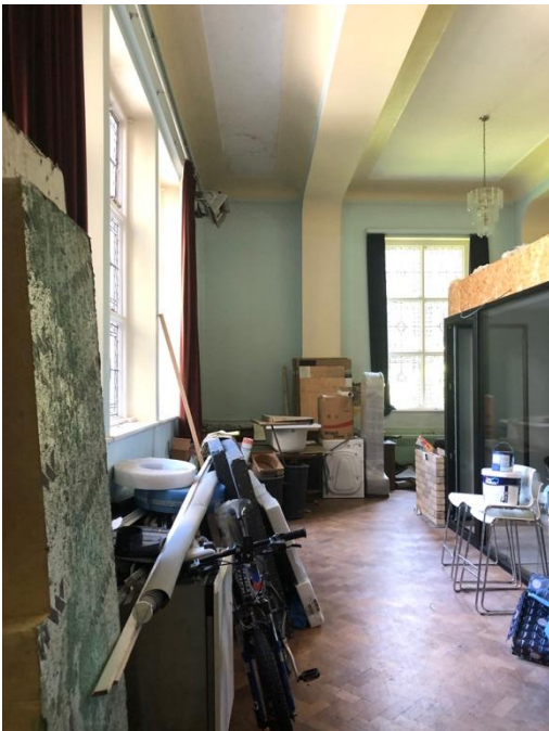
Plate 319: Grid structure within main room on upper floor level. Rectangular plan pillars support the beams spanning across the width of the room.
