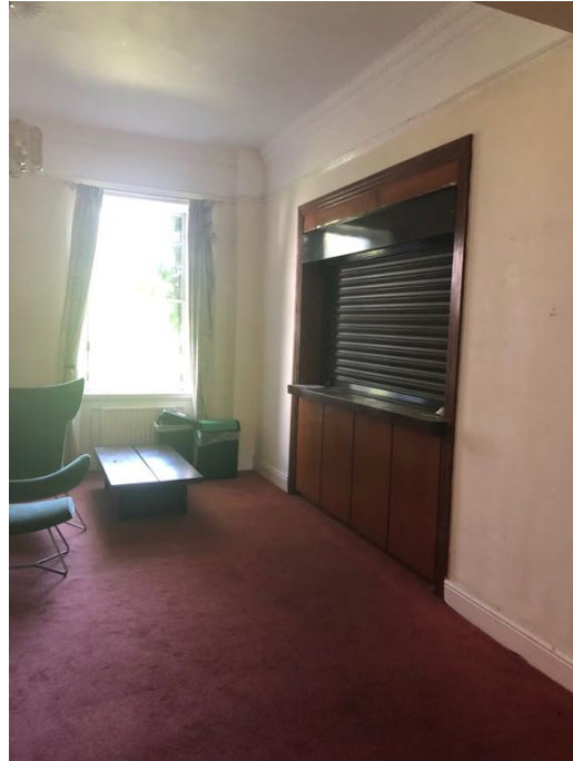
Plate 90: Sliding shutter to vestibule in same room
