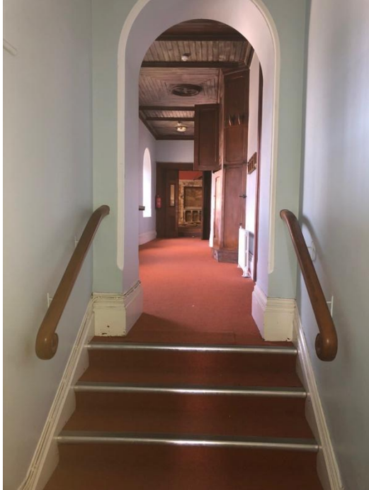
Plate 307: View along corridor on western side of complex between Building D (Chapel) and B2 towards chapel. Arch headed opening at connection to Building B2
