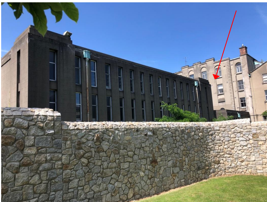
Plate 61: Southern elevation of Milltown house with Archive wing in context
