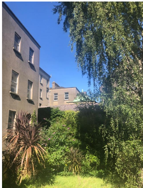
Plate 4: View west of the same elevation with the rear extension, link building and turret of small Sacred Heart Chapel (1911) in view
