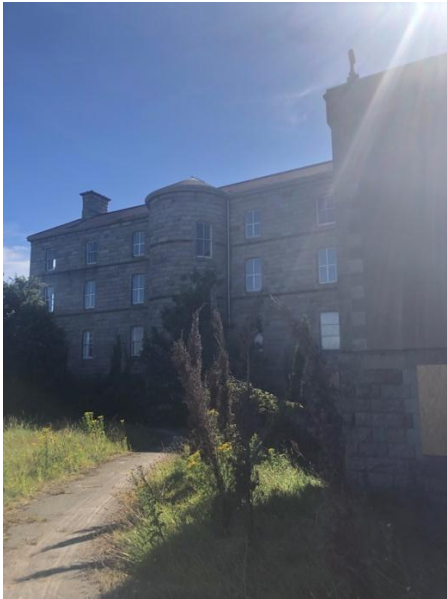
Plate 27: West elevation with bowed bay
