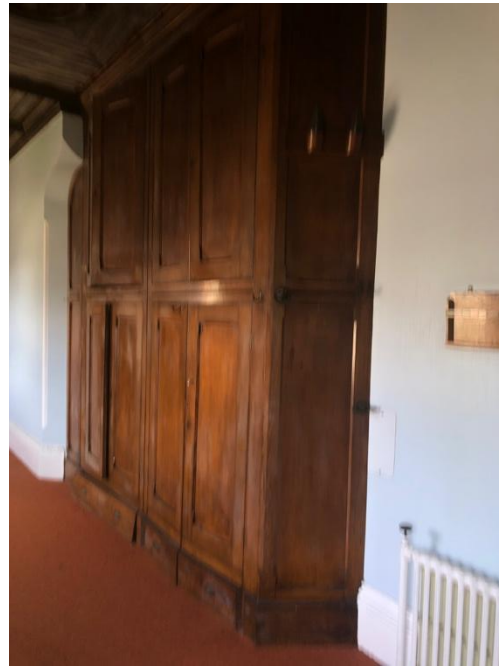
Plate 312: Panelled joinery within corridor linking Chapel to Building B2
