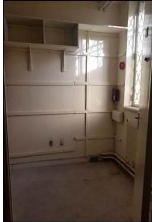
Plate 344: Large storage room
