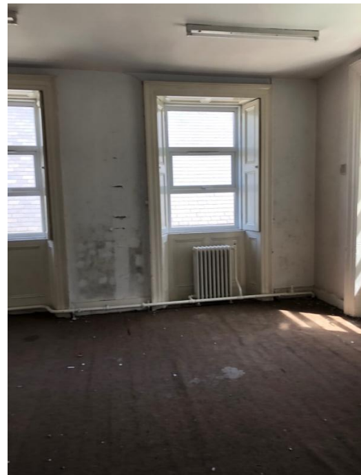
Plate 177: Larger office space
