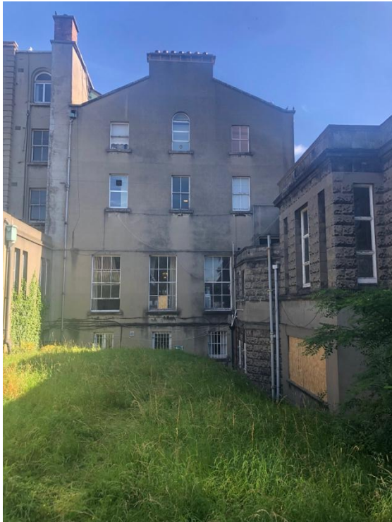
Plate 5: View of the much modified southern elevation of Milltown Park House where it connects to the Rear Extension, Finlay Wing and the Archive building
