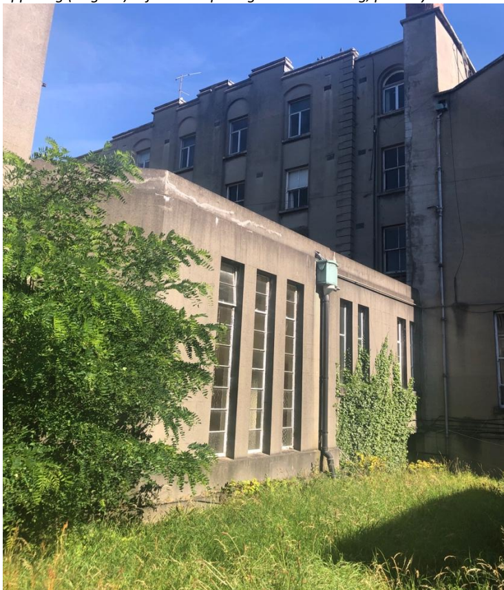
Plate 19: Southwest view of the rear extension, above the connection with the archive building.
