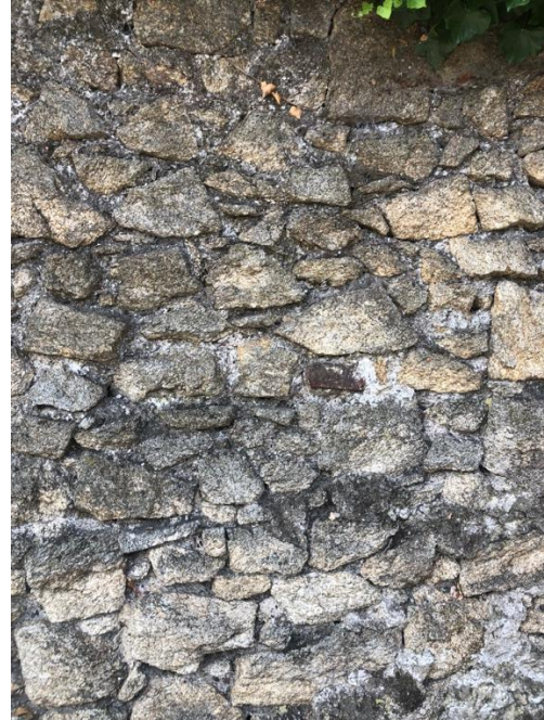
Plate 76: Composition of boundary wall varies, sections of rubble wall have been infilled
