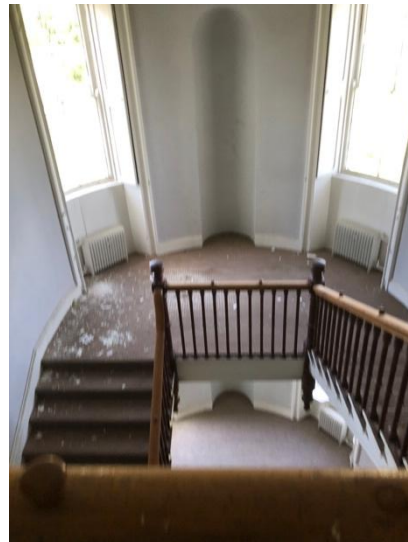
Plate 287: Level 2 landing facing north.
