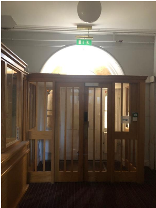
Plate 186: Later vestibule inside main entrance door.
