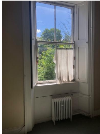
Plate 195: Two-over-two sash window, original shutters and architrave. Areas of plaster removed to reveal underlying masonry substrate.
