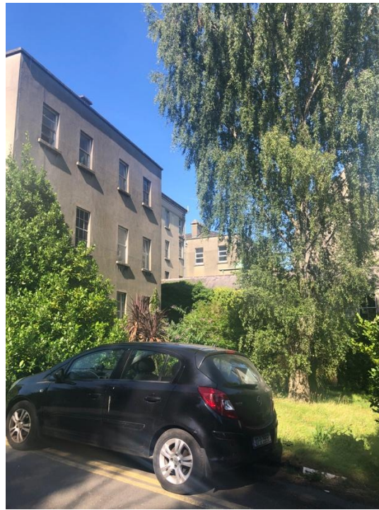
Plate 35: Link building connection to rear extension to Milltown house with small turret of Sacred Heart Chapel in view and larger domestic Chapel just out of view
