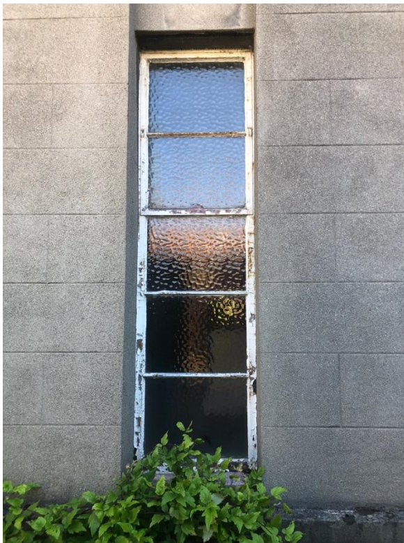
late 67: Detail of metal framed casement windows
