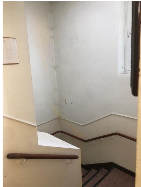
Plate 316: Contemporary stairs to basement.
