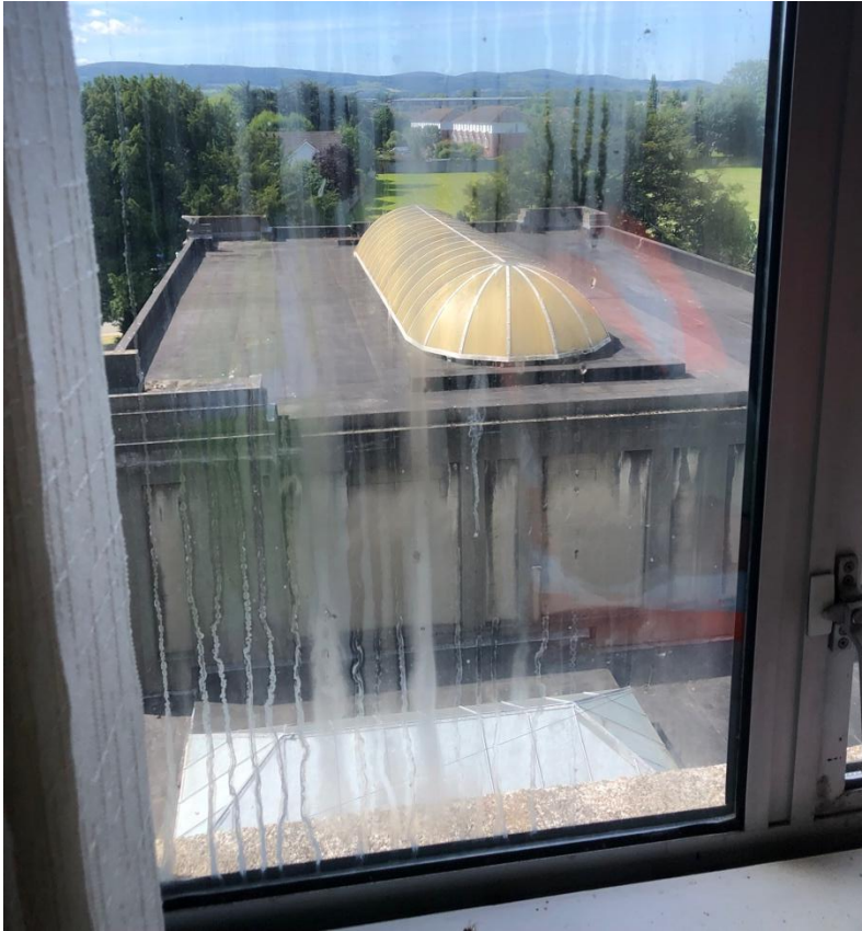
Plate 65: Roof of archive with domed roof lantern, as viewed from the rear extension to MPH
