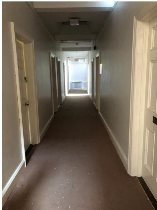
Plate 180: Central corridor at 2 nd floor level
