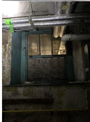
Plate 102a, b: 18 th century fabric within basement level accommodation
