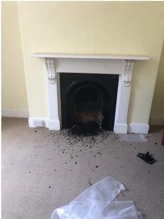
Plate 188: Corbel chimneypiece and cast iron insert
