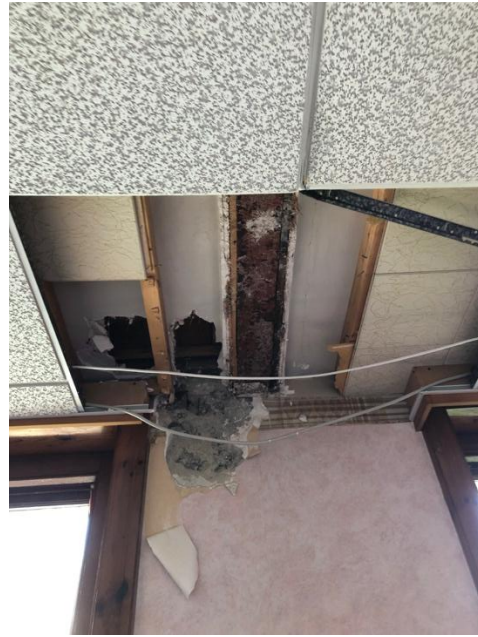
Plate 168: Multiple layers of past interventions Floor composition: floorboards on later timber joists, steel beams and 2 layers of later suspended ceilings.
