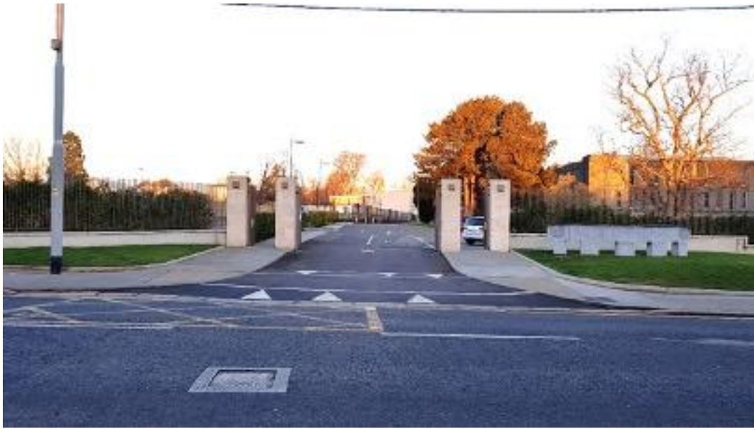
Plate 79: Entrance from Milltown Road
