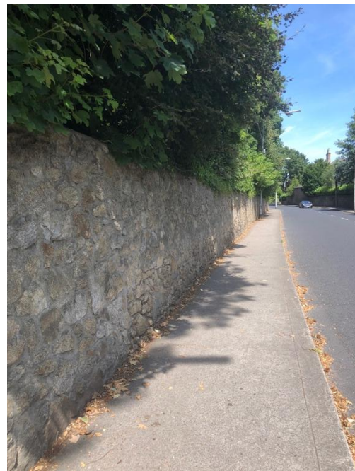
Plate 78: Curve of wall looking down Milltown Road, with pedestrian gate in centre
