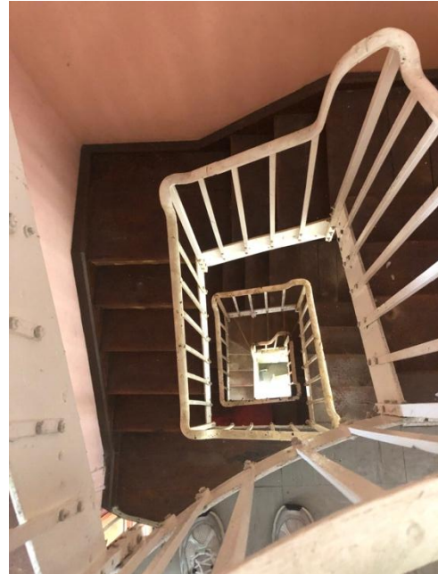
Plate 257: View down winding staircase
