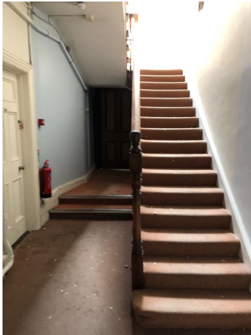
Plate 170: Stair at rear of block. Timber, open tread with turned bannisters.
