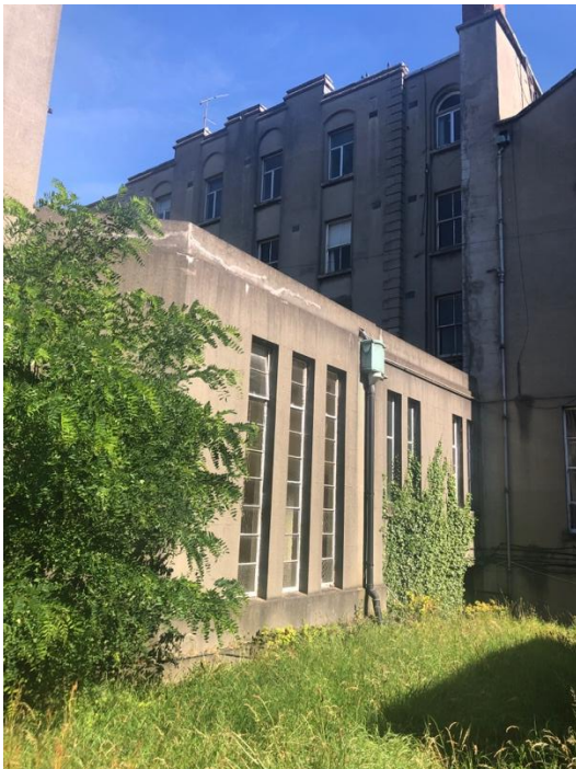
Plate 63: As above closer view of the Link to/from the Archive wing
