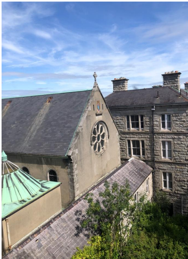
Plate 46: Roof of link building, facing towards south-west gable of Tabor House.
