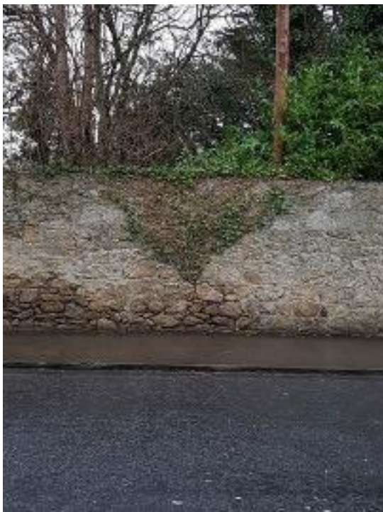
Plate 73: Section of rubble boundary wall on Milltown Road
