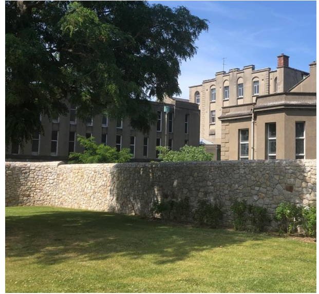
Plate 58: SE elevation, Finlay wing in foreground
