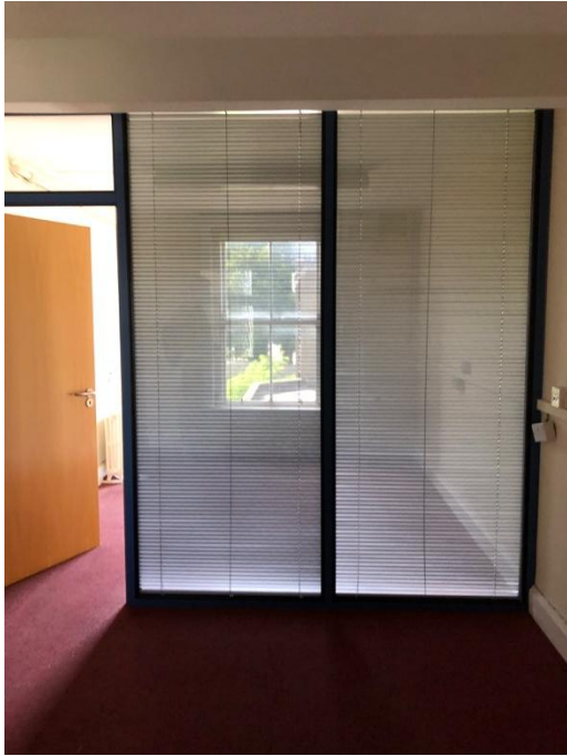
Plate 157: A typical dormitory with modern door
