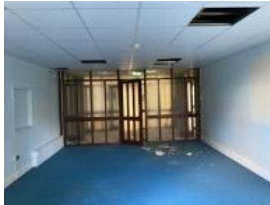
Plate 235: Later timber-framed fire screens within corridor.
