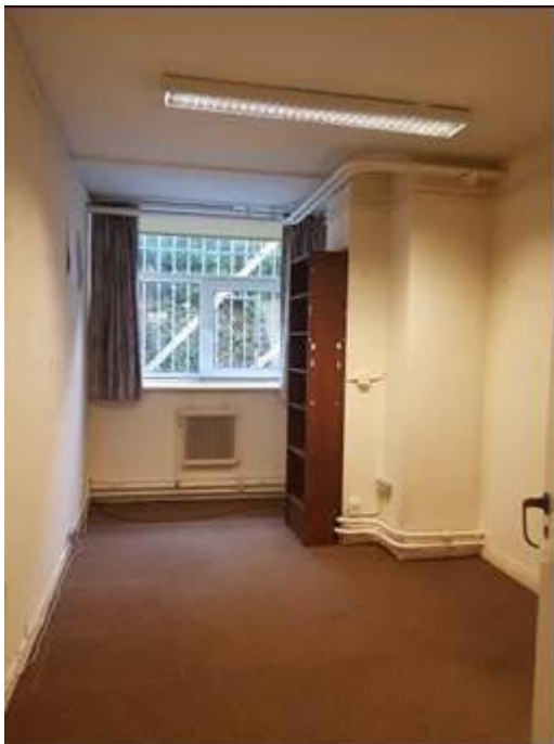
Plate 339: Lower ground floor level office within the Finlay Wing
