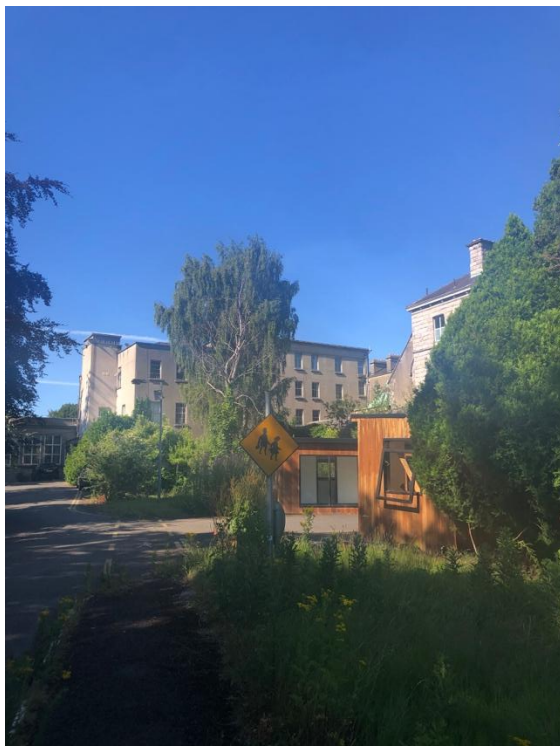
Plate 3: North east gable from drive way passing Tabor House (to right) with rear extension in context
