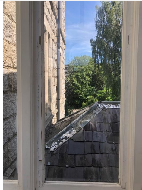
Plate 311: View east from window in linking corridor
