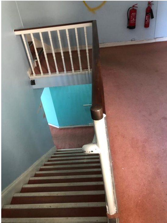
Plate 114:: Stairs from first floor viewing up
