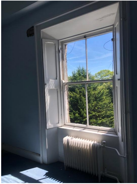
Plate 262: Second floor bedroom. Contemporary uPVC window frame with original timber window boxes.
