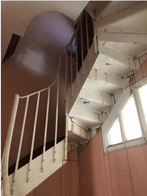
Plate 254: Secondary staircase in western bay with shaped flat metal handrail and square profile uprights. Vertical timber boarding to side of stair.
