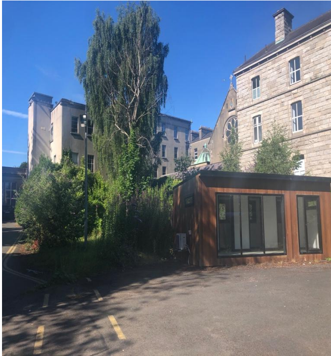
Plate 11: North east gable of rear extension block in context
