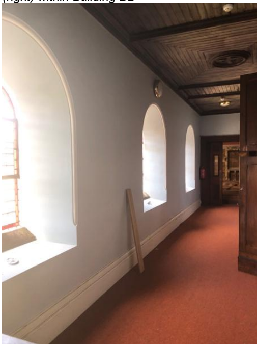
Plate 313: Panelled doors to Chapel, ceiling lined with diagonal timber sheeting.
