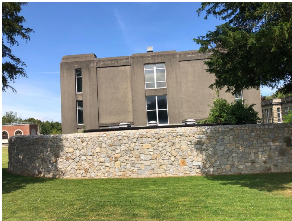
Plate 56: South-west gable of archive with 1970's single storey extension in foreground
