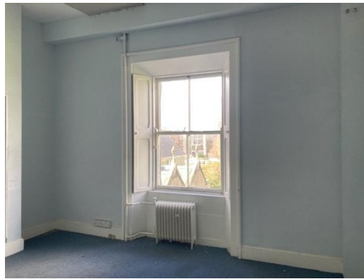
Plate 269: Original window box with contemporary uPVC window frame.
