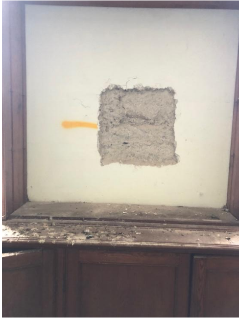
Plate 167: Opening up works reveal mix of technologies in the construction of MPH extension. Mass concrete walls in upper part of rear extension
