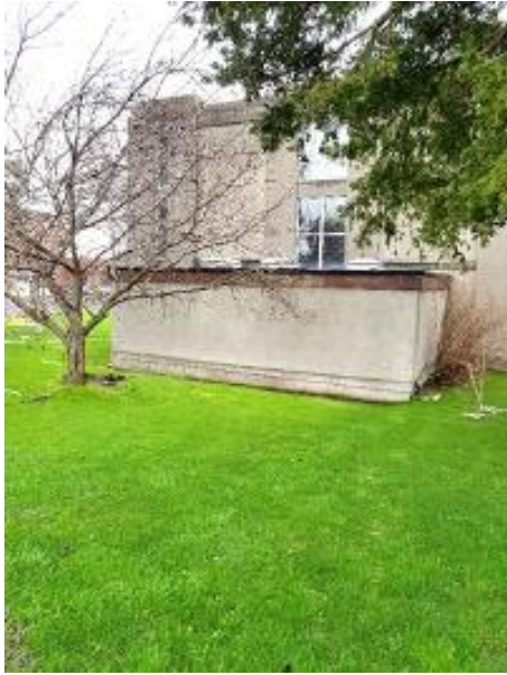
Plate 57:: SW Gable of archive
