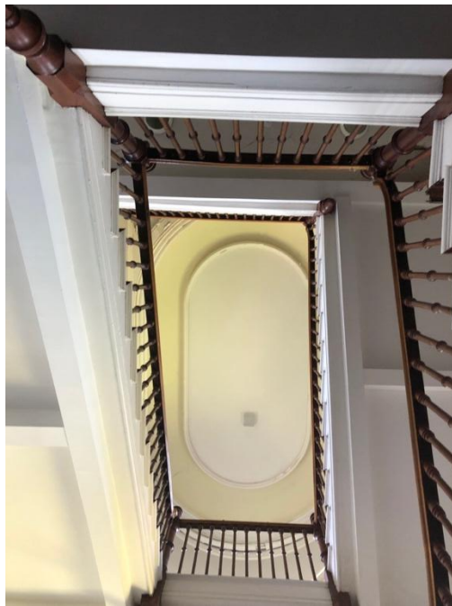
Plate 285: View up stair
