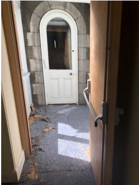
Plate 310: Link corridor to Chapel leading to choir stalls in the gallery area. Round headed panelled door with glazed upper panel.
