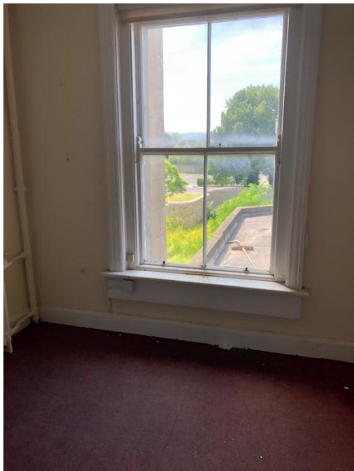
Plate 182: Typical small lecture room absent of decorative detailing and having modern window at second floor level
