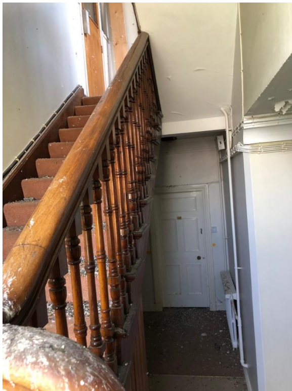
Plate 172: Detail of stair from 2 nd to 1 st floor
