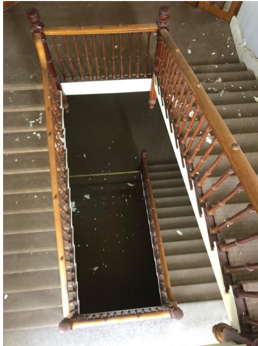
Plate 283: View down central stair
