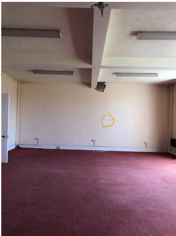
Plate 144: Exposed structural grid in rear extension.
