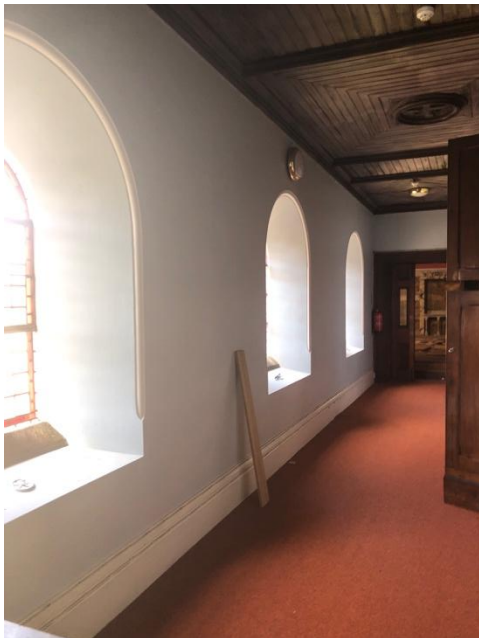
Plate 309: Detail of timber panelled ceiling.
