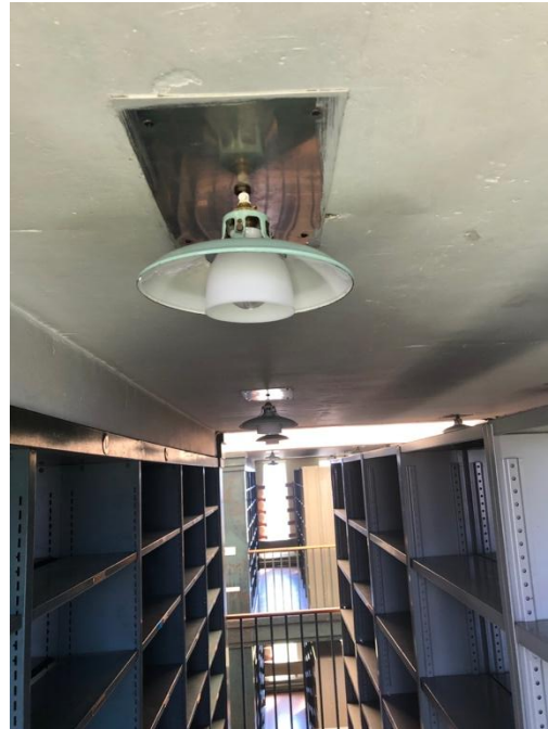
Plate 360: Example of light fitting common throughout
