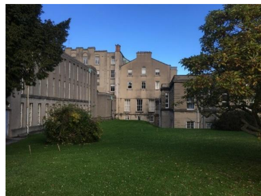
Fig. 24 Southern elevation, comprising an extension, with its expressed gable. Note the uncomfortable connection with its rear, later, extension, at a storey higher.
