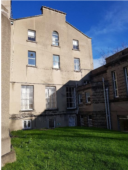
Fig. 25 Southern elevation, comprising an extension, with its expressed gable in context with the Finlay Wing and Archive (corner visible). Lower windows are early in origin, with the 6/6 windows attached to a former orangerie, which was vertically extended in the 20 th century.
