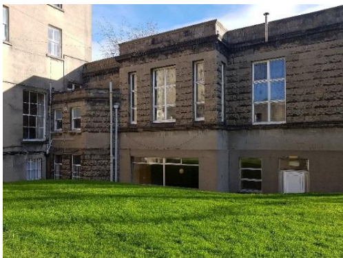
Fig. 46 View of west elevation
