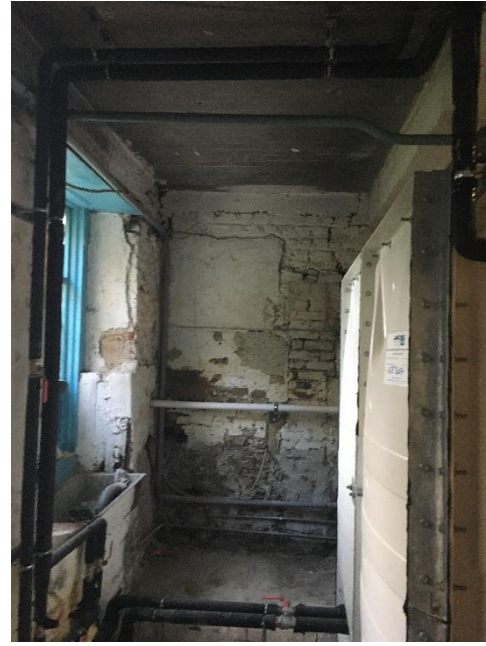
Fig. 34 View east in same room
