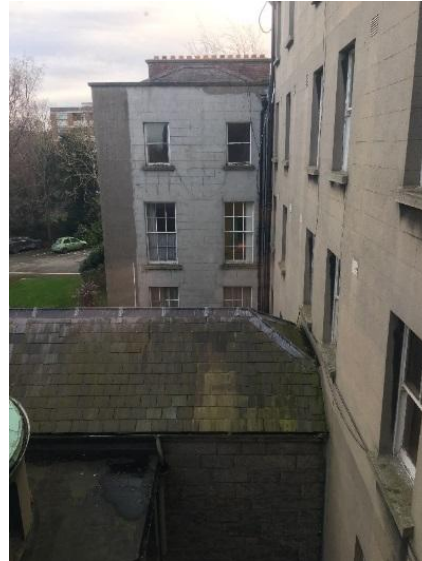
Fig. 26 Part of rear (west) elevation, with uppermost level added, and in context with its higher rear extension.
