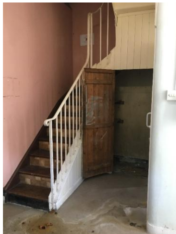
Fig. 70 Secondary steel stair of interest
