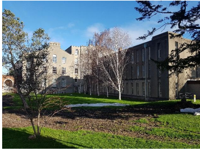
Fig. 56 West elevation in context with Extension Block
