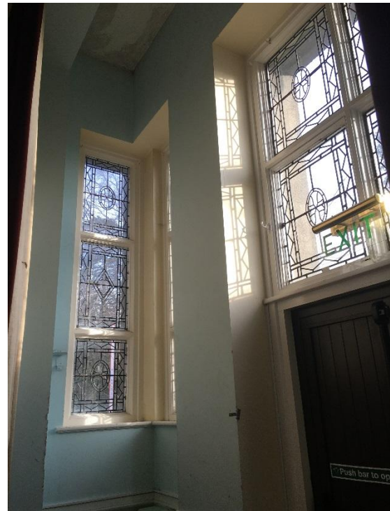
Fig. 49 Leaded windows within lobby to east
