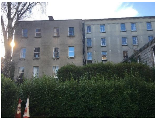
Fig. 36 The extension's later northern infilled section in context with the north elevation of the main house, with the two storey Chapel link to the RHS of the image.
