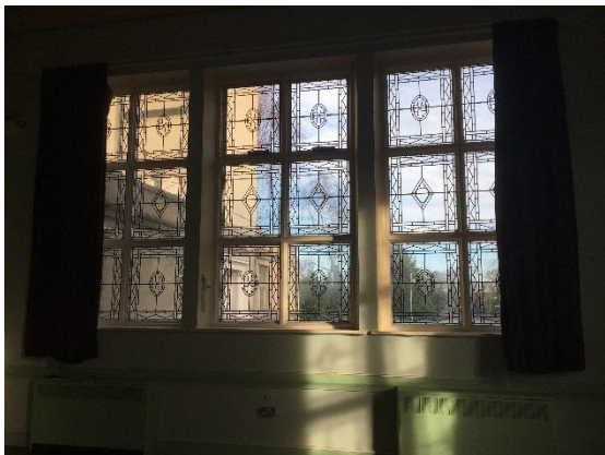
Fig. 50 North elevation leaded window
