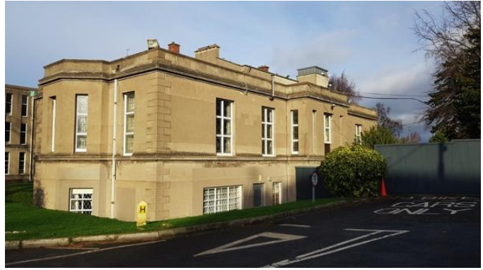
Fig. 44 View of east elevation
