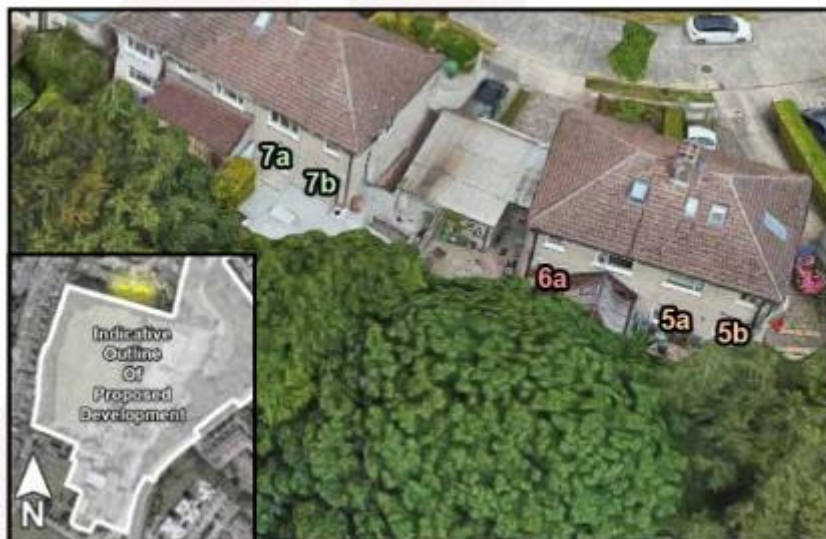
Fig. 5.5: Affected windows Norwood Park.
