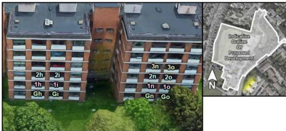
Fig. 5.4 Affected windows on Rowan Hall / Cedar Hall (L) Aerial view of assessed locations (R)
